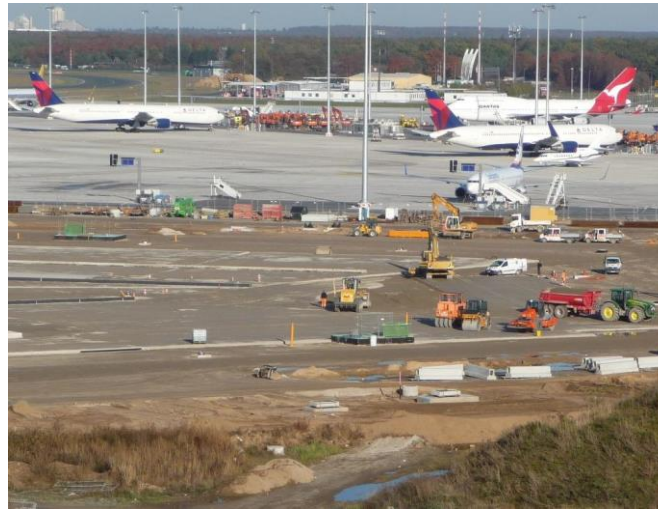
Frankfurt Int. Airport – Ramps 4 + 5 Masses approx. 180.000 m 3 , Concrete/Asphalt surface approx. 188.000 m 2
